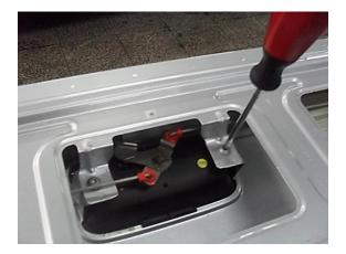
3) Install the base plate and actuator kit, hold in place by replacing the removed screws from no.3
